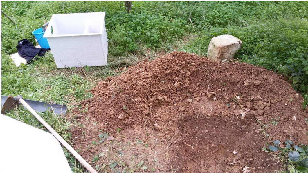
Figure 1: An area was dug out to make space for the silt trap which needs to be at ground level to allow the flow of rainwater into the silt trap.
