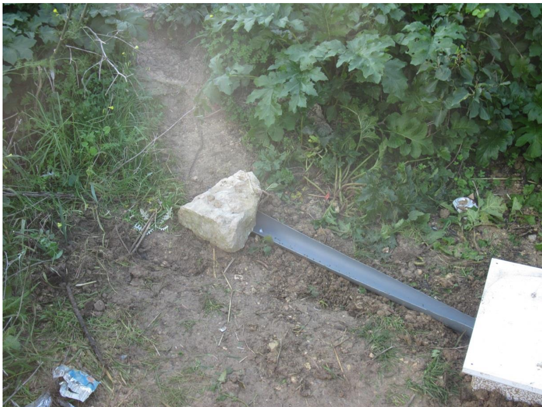
Figure 3: The gutter was moved to a position in order to improve the flow of water and avoid water from being diverted away from the gutter.
